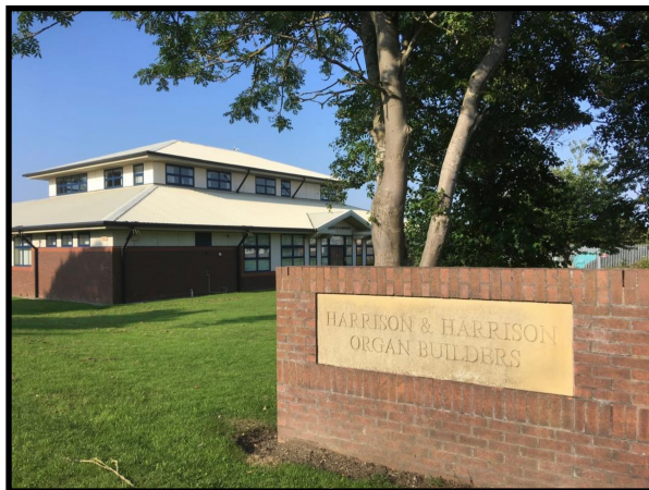
The modern premises of Harrison & Harrison, Durham.
